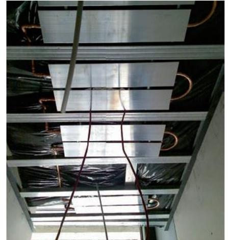
The heated/chilled ceiling elements are located behind a perforated suspended drywall ceiling
