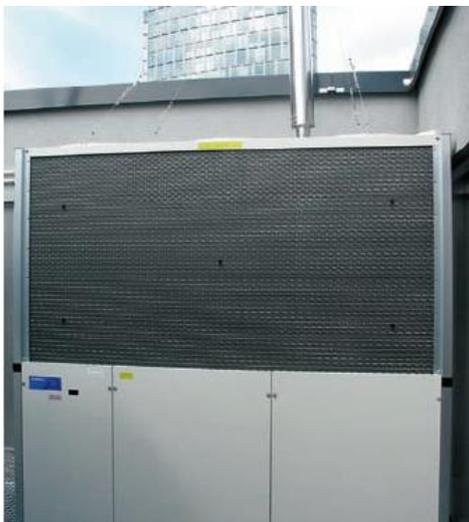
Three natural gas-operated reversible heating pump/cooling machines are used for the generation of heating and cooling performance at the Westpol building (installation on the roof)
