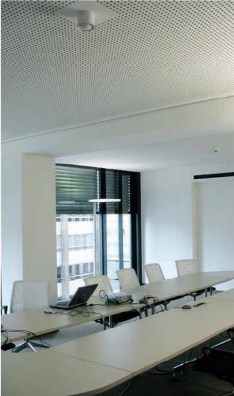
In the Westpol building, all of the office and conference rooms are equipped with combined heated/chilled ceilings and are supplied with conditioned supply air
