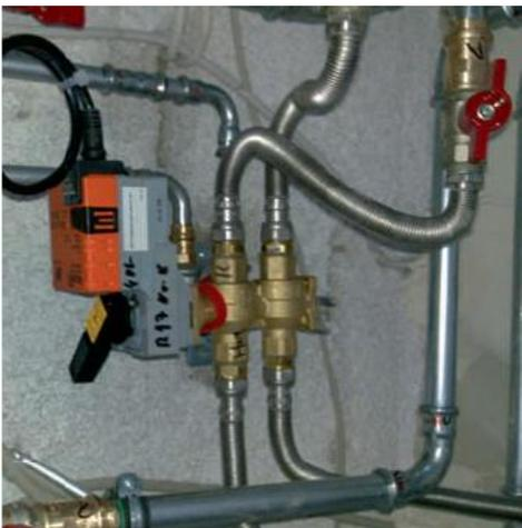
A 6-way characterised control valve (CCV) after installation (behind a suspended ceiling in the corridor area)
